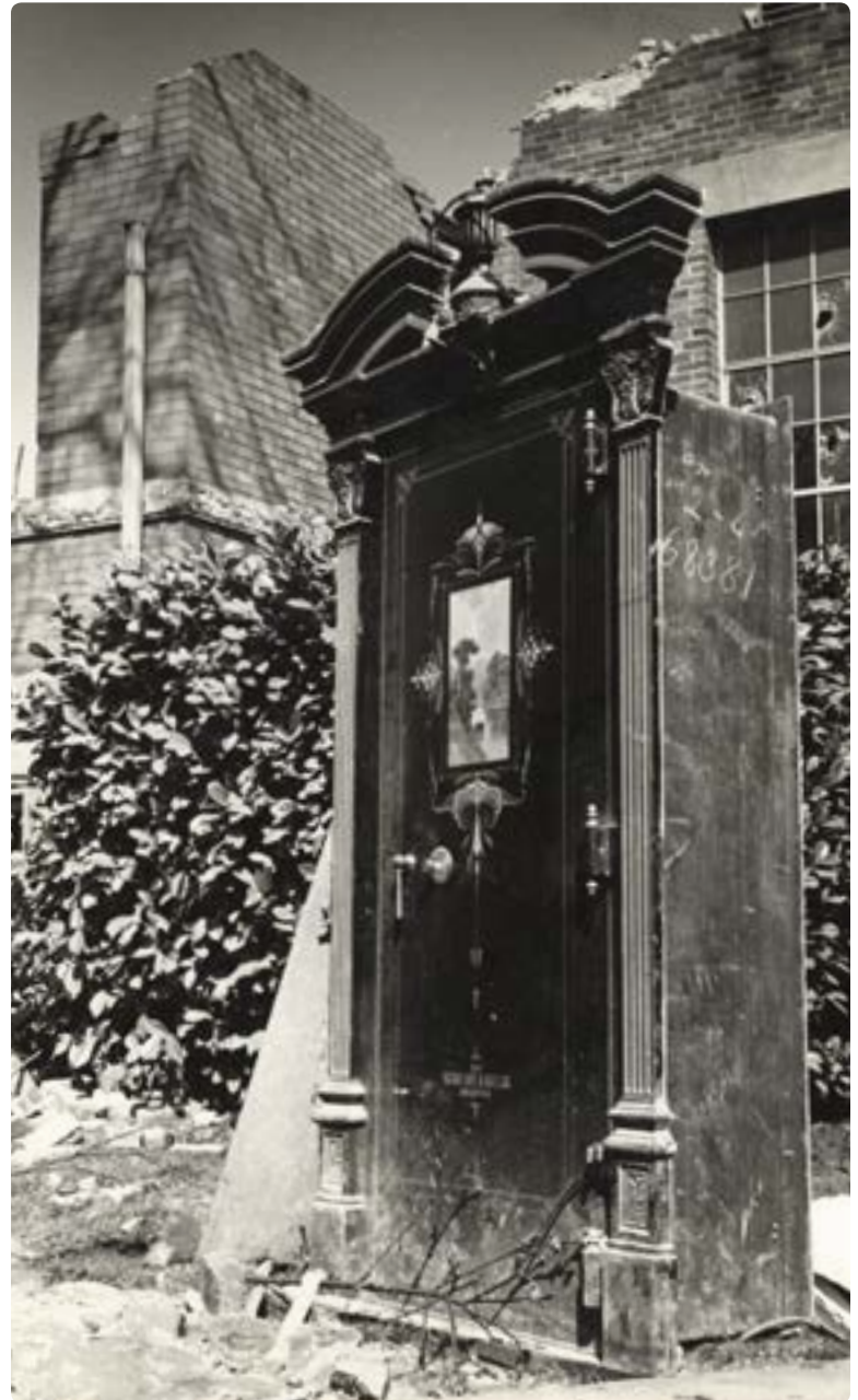
Right: GN7400, Vault door for the Lane County Clerk's safe, removed from the 1898 Lane County Courthouse when it was razed in 1959.
